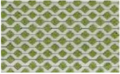
Grass Pavers Combines greenery with functional load-bearing surfaces; reduces surface heat, supports infiltration
