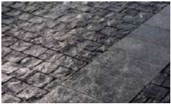
Natural Stone Pavement Locally sourced & textured, suitable for high-traffic pedestrian areas; Reduces thermal gain, blends with softscape
